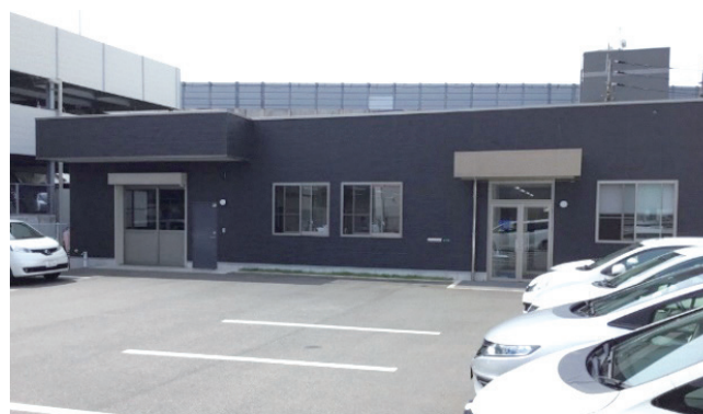
SMC Corporation's Kitakyushu Sales Office (outside view)
