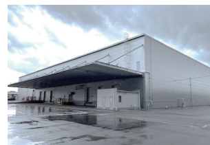
NX Kumamoto Logistics Center (outside view)
