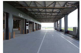
NX Tosu Logistics Center (road inside building)
