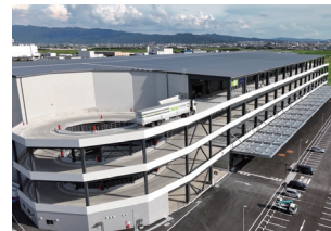
NX Tosu Logistics Center (outside view)
