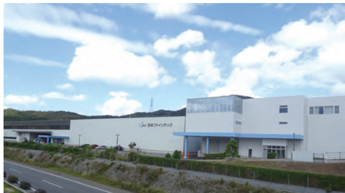
Panoramic view of Miyawaka Plant
